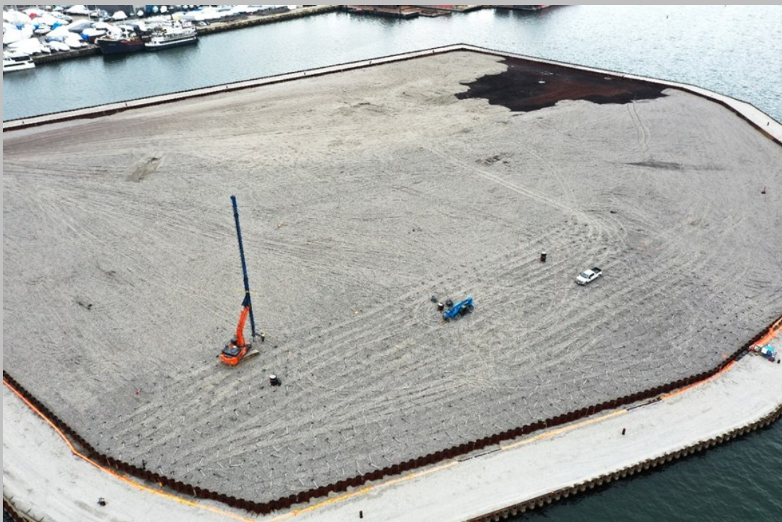
Wick drain installation within 1/4 of the drainage stone.
