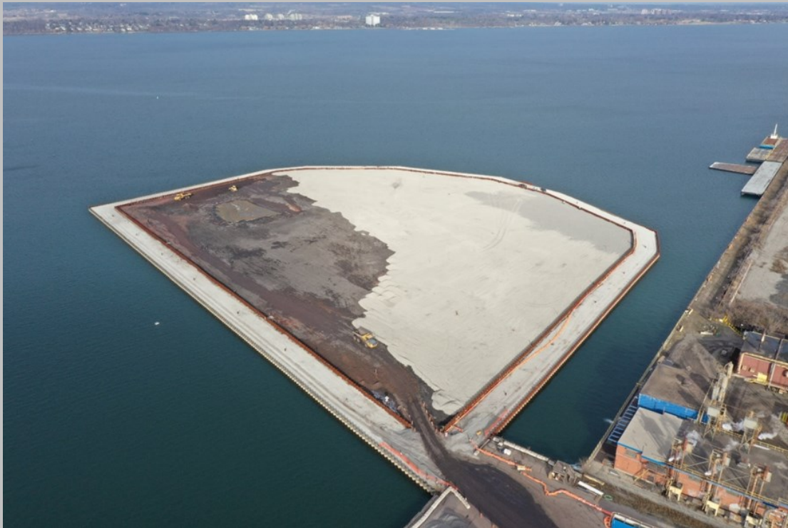
Drainage stone installation completed on 2/3 of the ECF surface.
