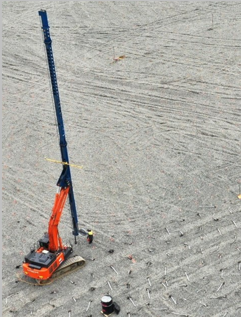
Detail of wick drain installation.
