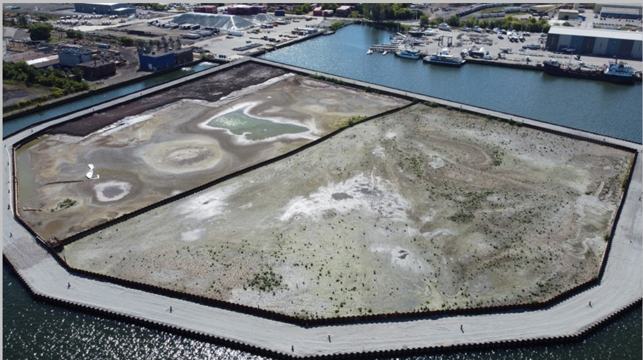
Aerial view of the ECF in September 2022
