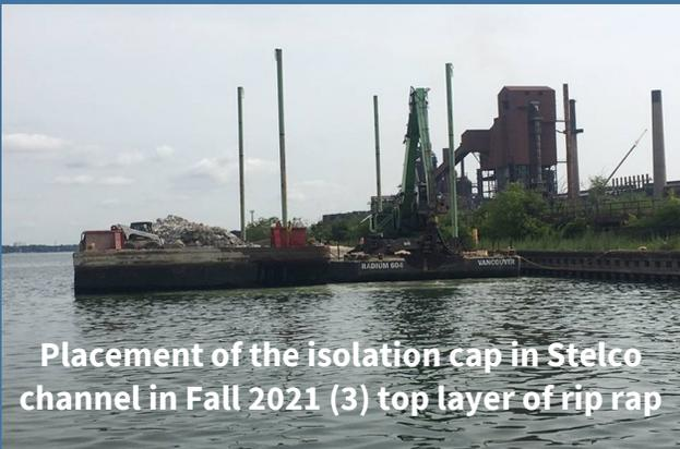
Placement of the isolation cap in Stelco channel in Fall 2021 (3) top layer of rip rap
