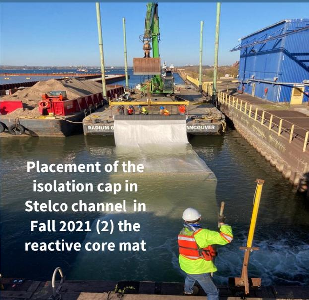
Placement of the isolation cap in Stelco channel in Fall 2021 (2) the reactive core mat
