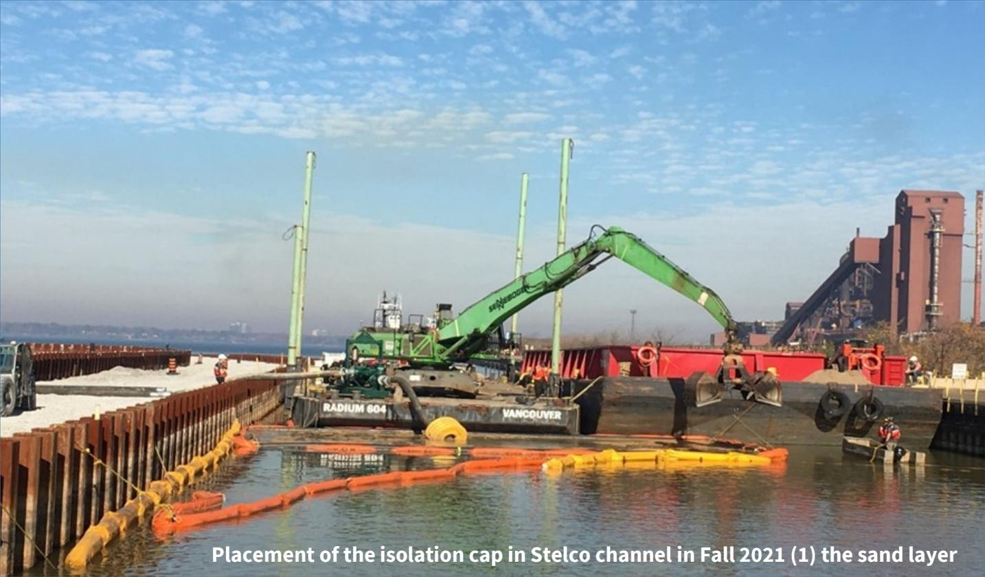
Placement of the isolation cap in Stelco channel in Fall 2021 (1) the sand layer
